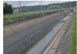
State of a waterway 19 years after frost damage repairs were conducted.
